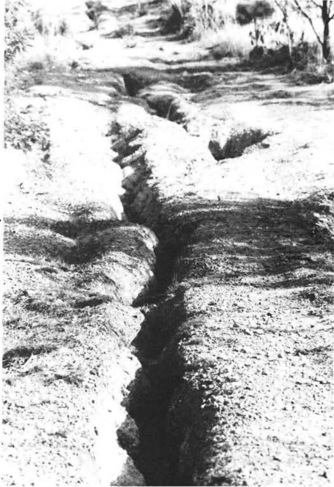
Rill and tunnel erosion along a four wheeled drive track at Government Hills near Risdon Vale.
